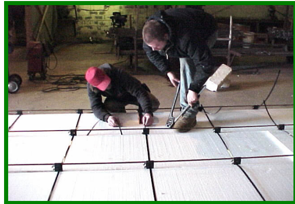
Figure 10 Prefabrication of EPS Panels
