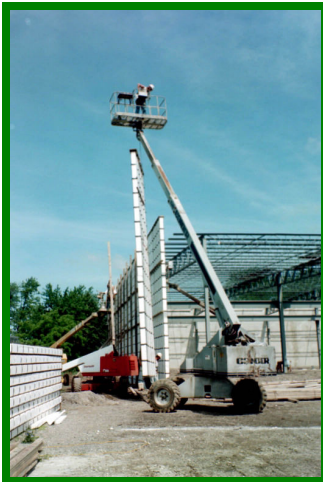
Figure 14 Boom Lift Maneuvering an EPS Panel into Place
