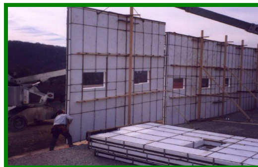
Figure 15 Anchoring Panels to Footers
