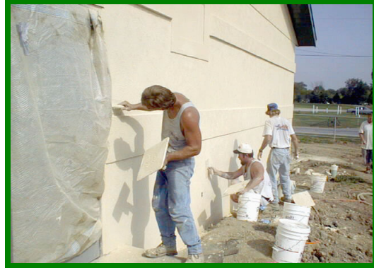
Figure 18 Finishing of Shotcrete Surface
