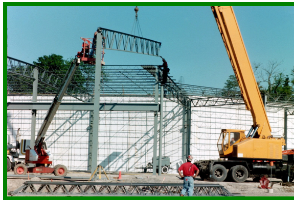
Figure 12 Erection of Structural Steel Support Frame
