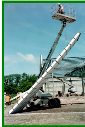
Figure 13 Boom Lift Tilting-up an EPS Panel
