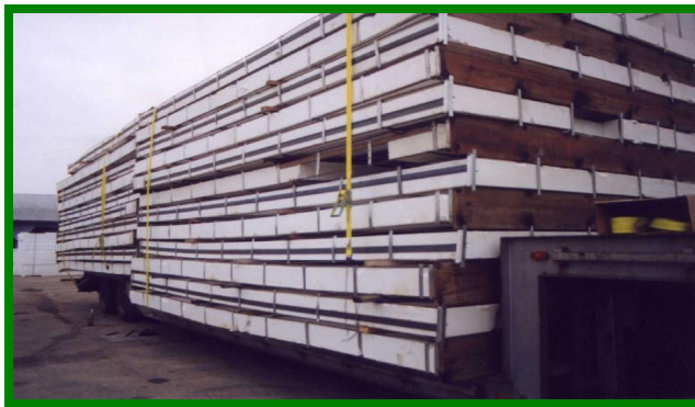
Figure 11 Prefabricated Panels are Loaded for Delivery to Jobsite
