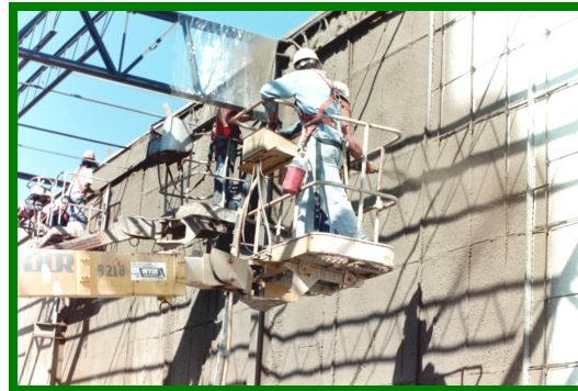
Figure 17 Application of Shotcrete
