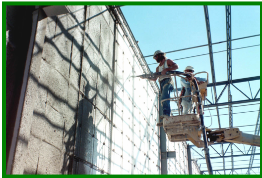
Figure 16 Application of Shotcrete
